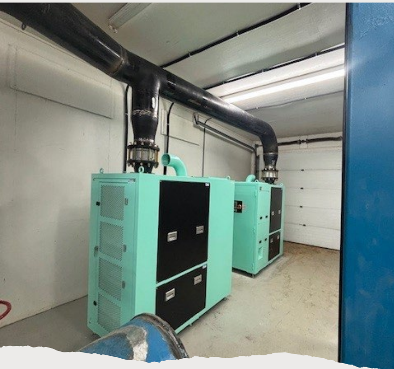
New High Efficiency Blower Installation (to be commissioned this week)
